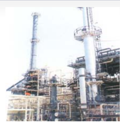
Shell Brunei Refinery Construction
