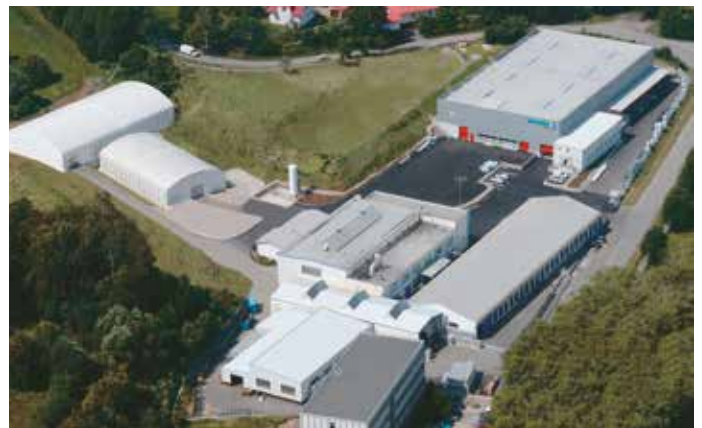
Plant Ledec nad Sázavou (CZ)
