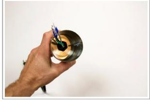
2. Remove the nut and washer from the bolt, and slip the green ground wire spade connector over the bolt. Slip the stainless washer over the bolt and retighten the nut. Use a plier and your robertson screw driver to firmly tighten the ground to the element enclosure.
