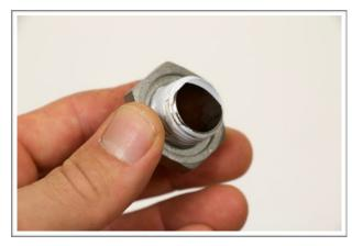
3. Thread the pipe nipple into the ball valve on the same side that you threaded the locknut. Finger-tighten it for now. The groove for the silicone washer should be facing away from the ball valve.
