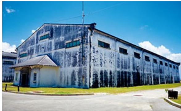
The black stuff that you can see on the walls of the warehouse is the ethanol-loving Baudoinia mould.
