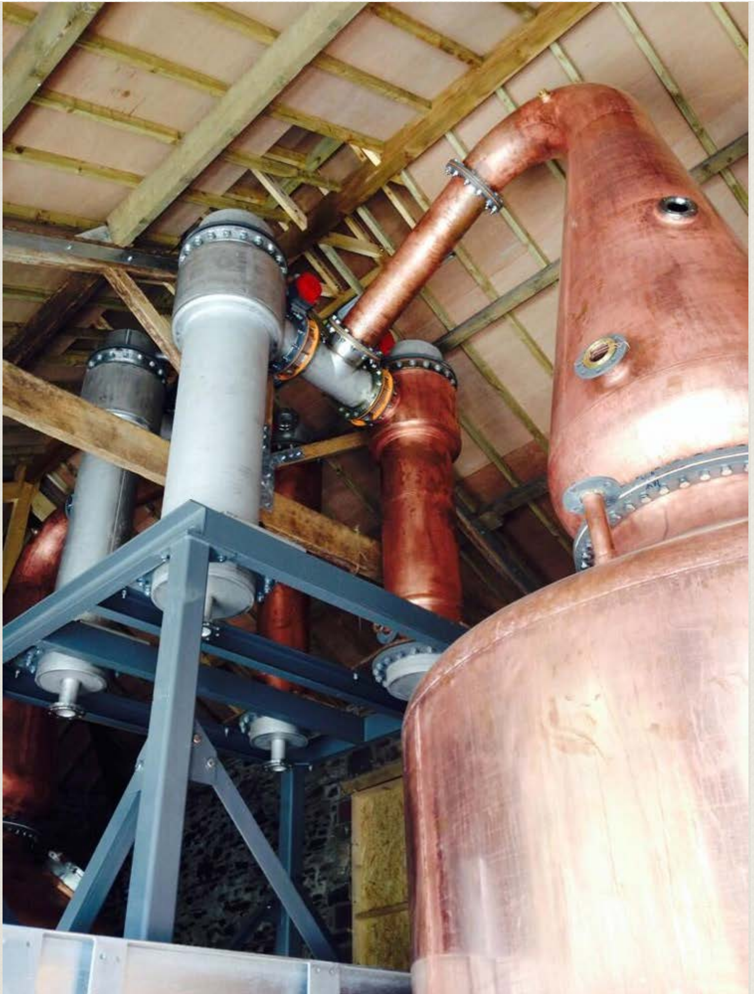
Double shell and tube condensers at the Lakes Distillery.
