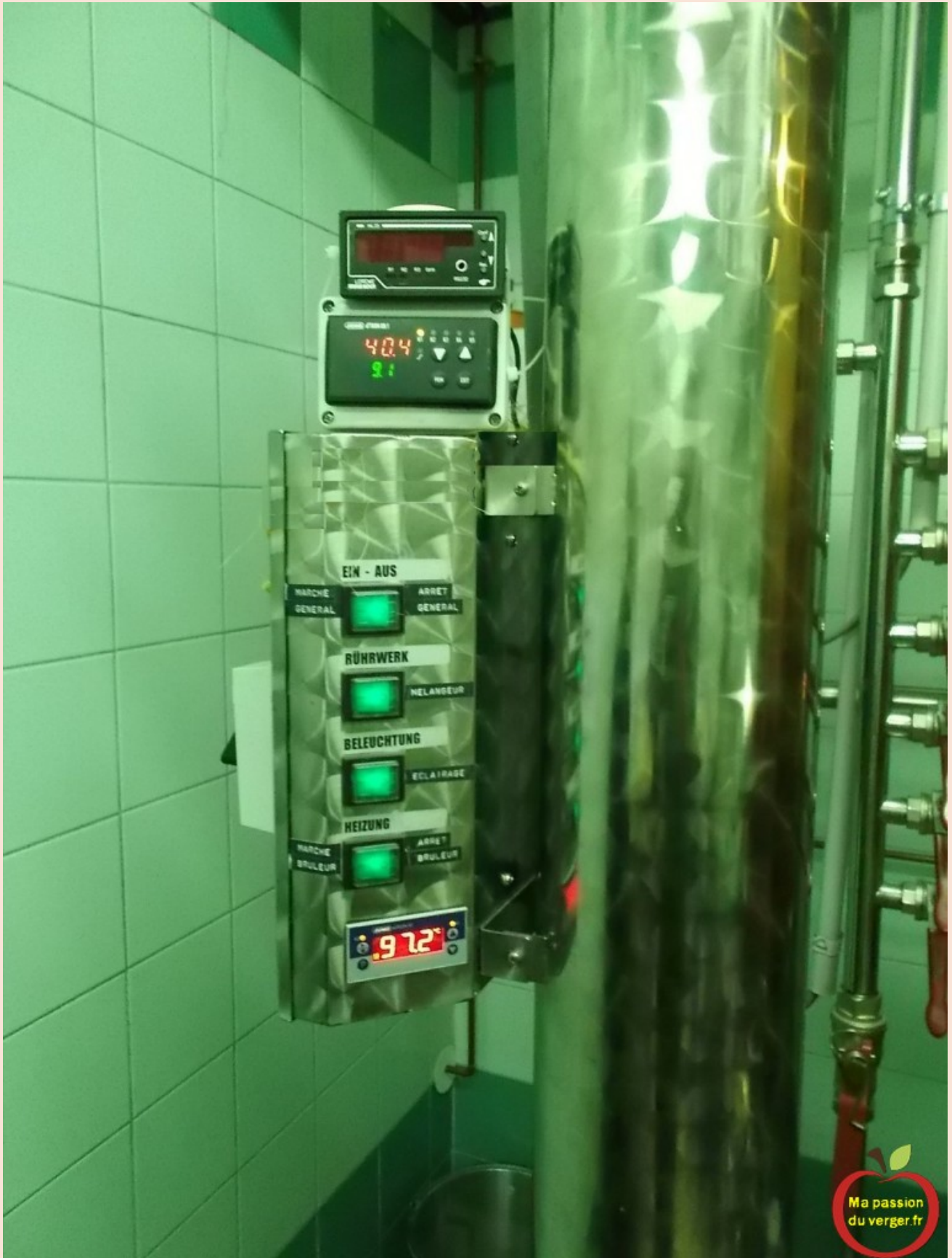
Commissioning of the control box.
