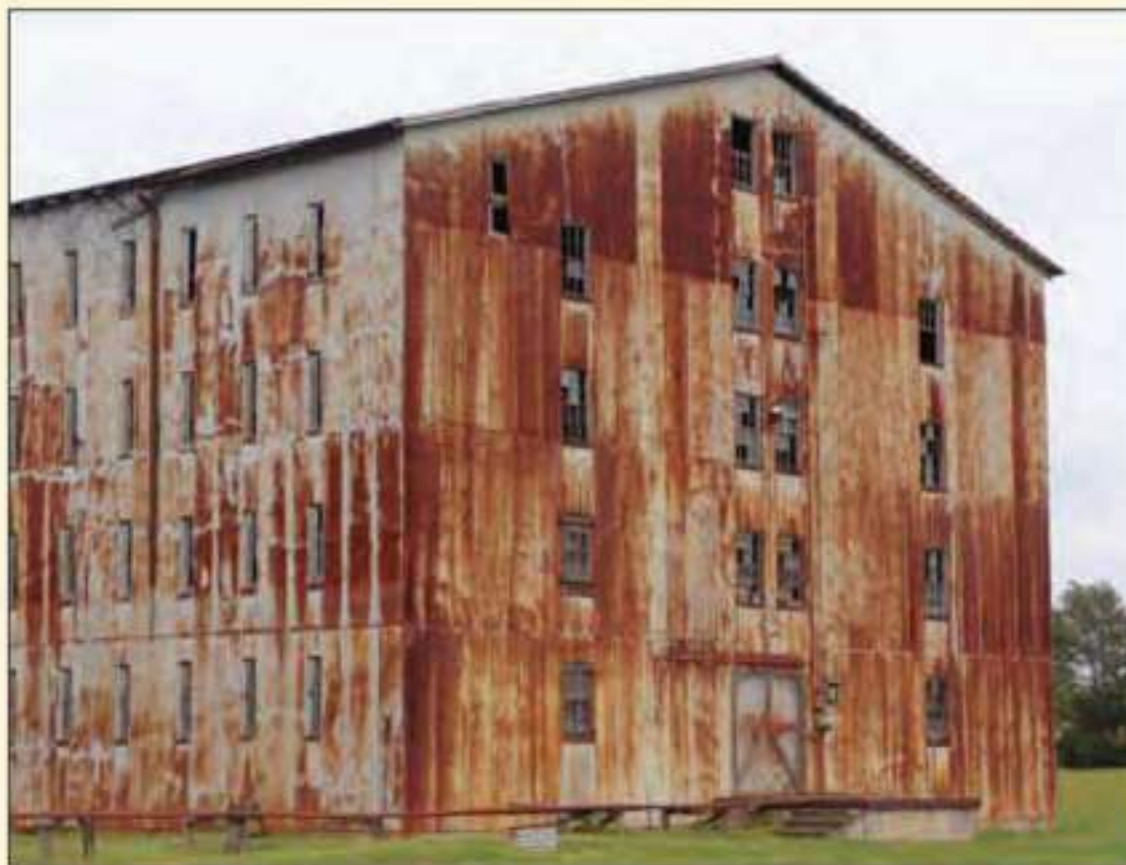
In this whiskey barrel storage building, a black mold and rust thrive on the “angel’s share” of evaporated alcohol and the Kentucky humidity.
